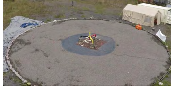
Landing Pad Pavers
